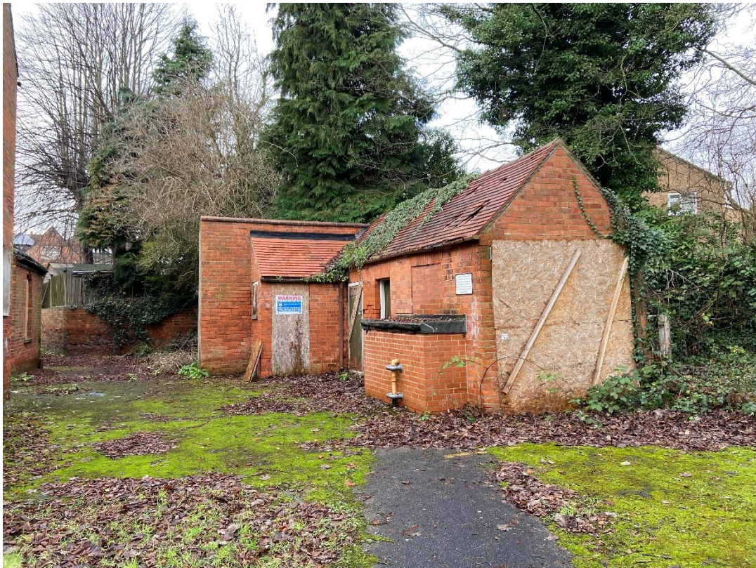
Outbuilding to be demolished with 30-32 Sewell Road in background to right
