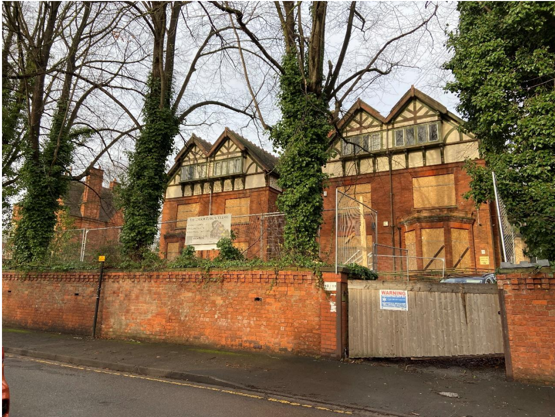
Front elevation with 9 Lindum Terrace in background
