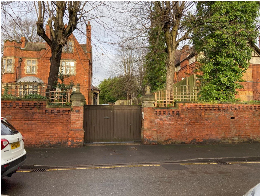
Front elevation and access to be widened
